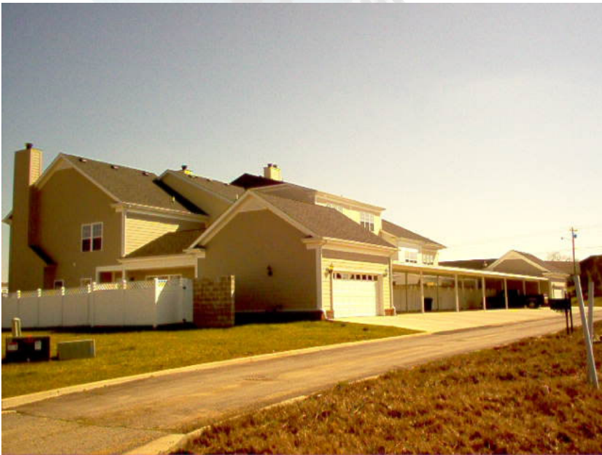
Rear - 8 Unit Bldg
