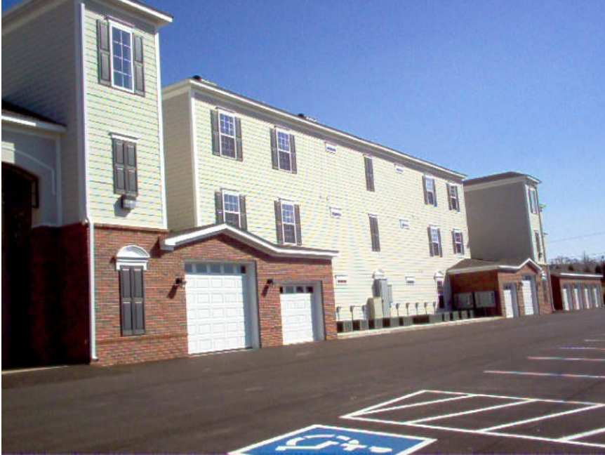
Rear - 24 Unit Bldg
