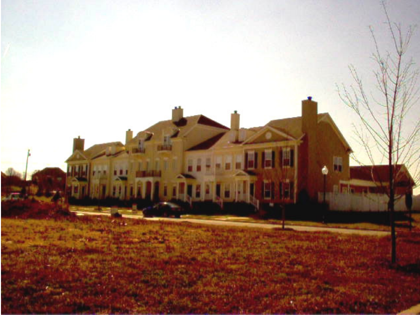
Front - 8 Unit Bldg
