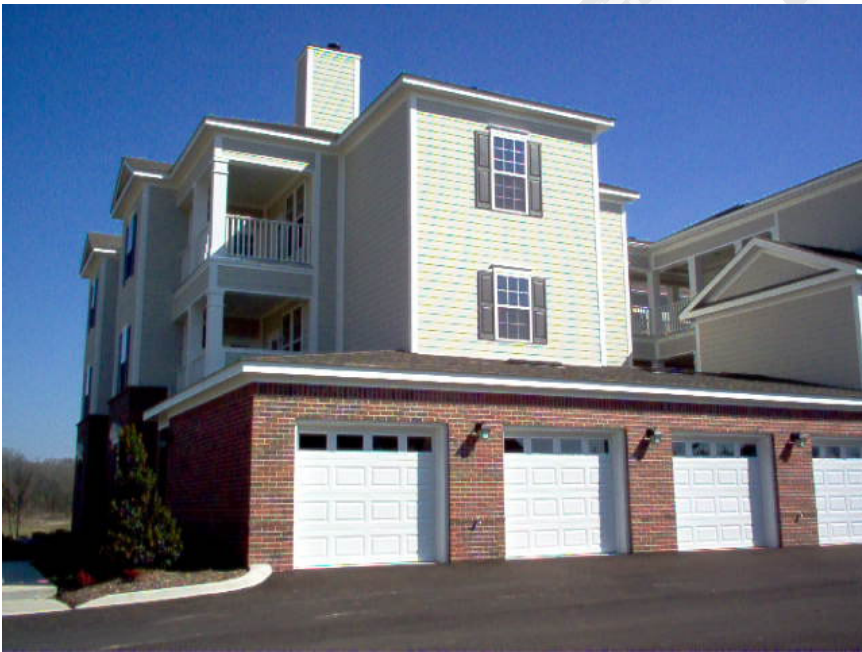
Side - 24 Unit Bldg
